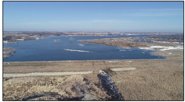
Upper Maple River Dam – Maple - Steele County Joint WRD
